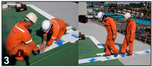
Unroll, peel back release sheet, align, press and step down hard on DrySeal hatch tape is fully adhered to the surface. Cut into required lengths if required.
