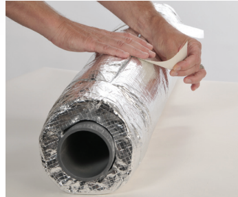
3. Remove inner layer of exposed Tape and press Tape to secure.
