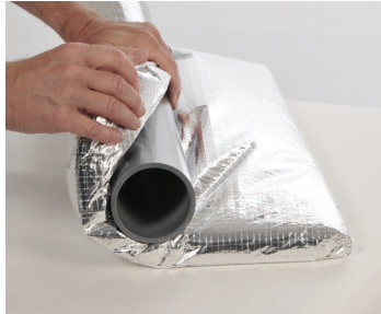
2. Wrap material around Pipe.
